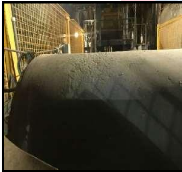
Figure 2. Condition of Previous Belt - Worn Out Belt
